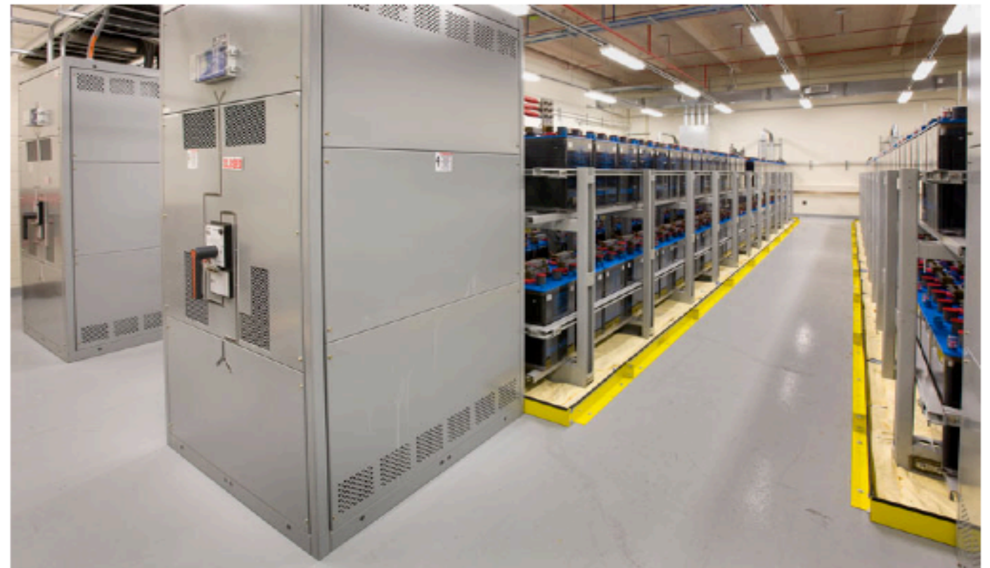
Lead Acid Data Center Battery Room
