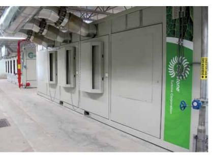
A natural gas and methane gas fueled Capstone C1000 and CR600 at York's wastewater treatment plant save energy, cut operational costs and protect the environment by generating clean-and-green electricity.
