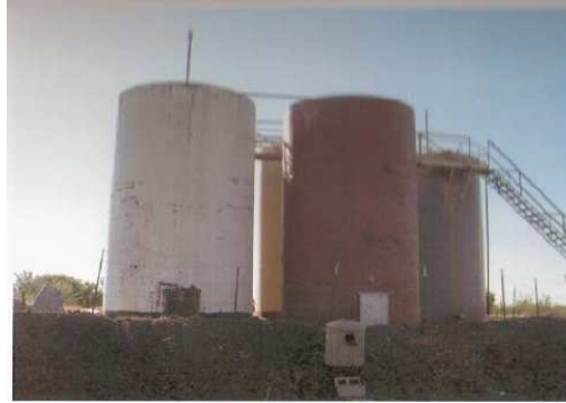
Photo No. 1 – Patrick Welder Tank Battery
