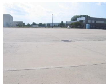
Figure 2: Deicing Pad with Drain
